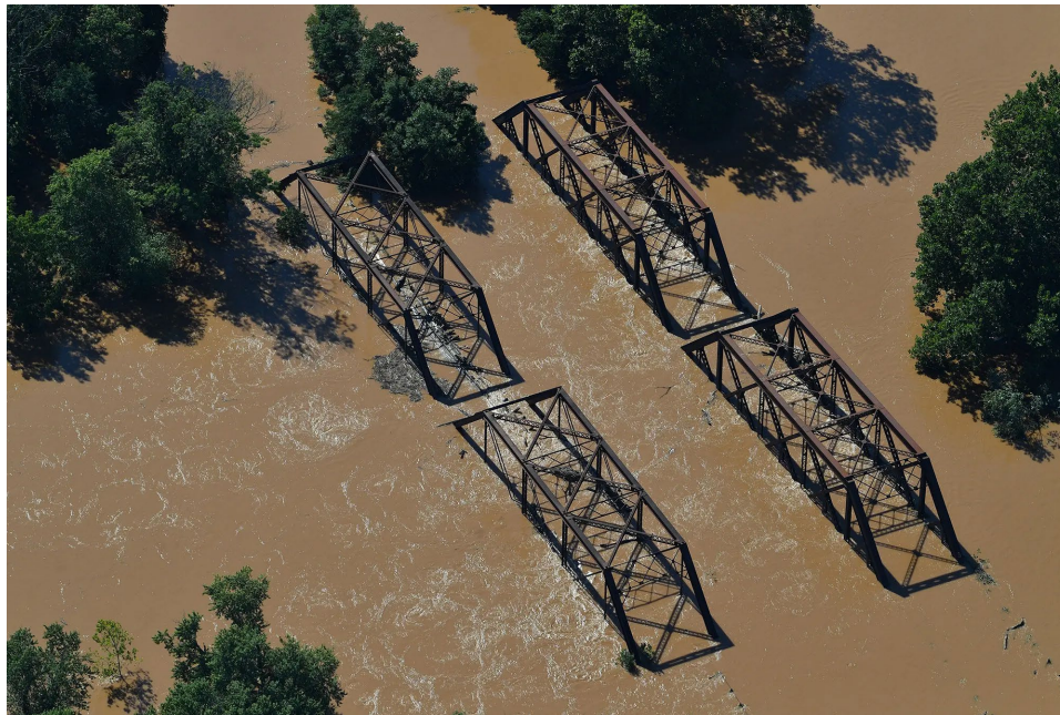
Figure 15 : Bridge in Somerset County Inundated by Floodwaters
